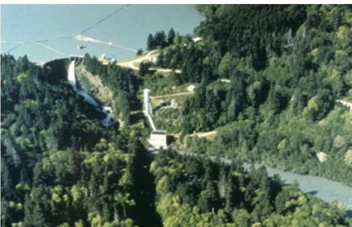
Glines Canyon Dam before removal
