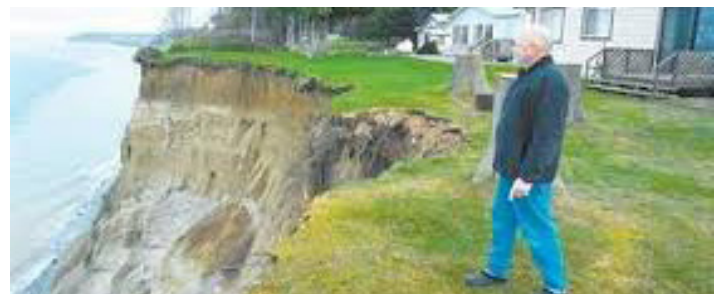
Bluff erosion in Clallam County
