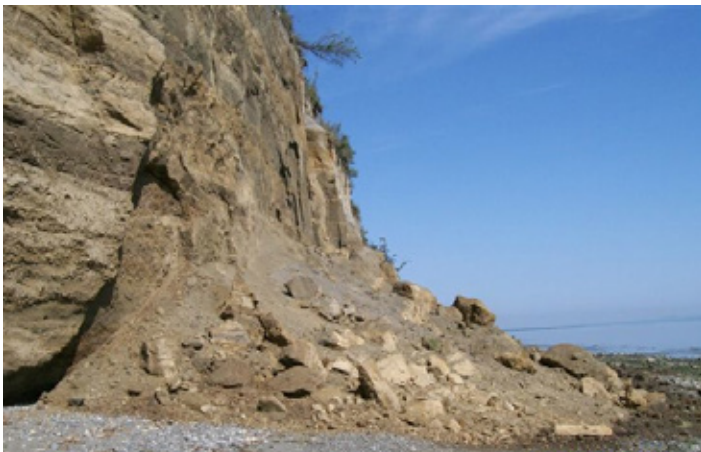
Eroded Bluff on Clallam County Coastline
