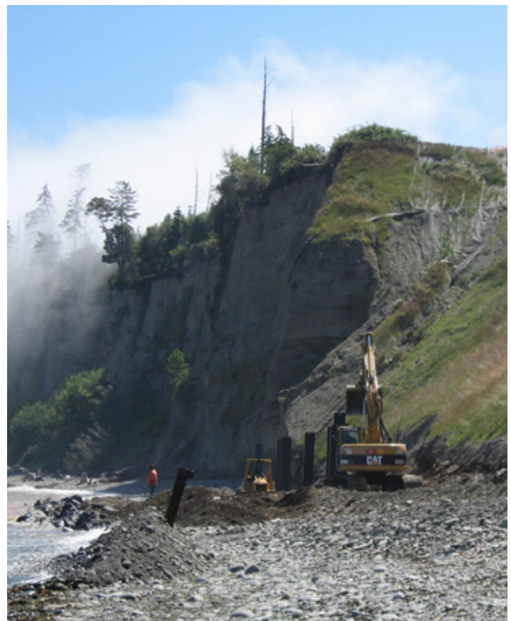
Port Angeles Landfill Seawall during construction, 2007
