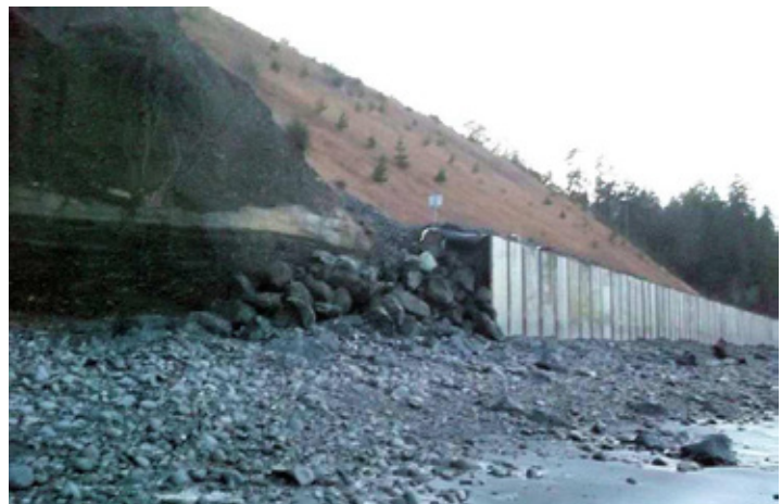
Completed seawall-Port Angeles Landfill
