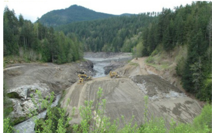
Elwha Dam Removal, 2012
