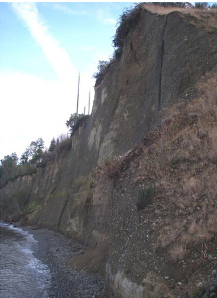
Current site conditions east end cell 304
